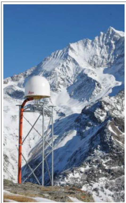
Figure 6. Rock movement detector and station.
